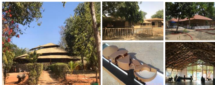
Figure 31 Construction of building prototypes (Source: Author)
